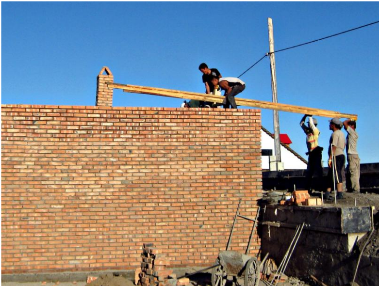
The construction of the water supply station
